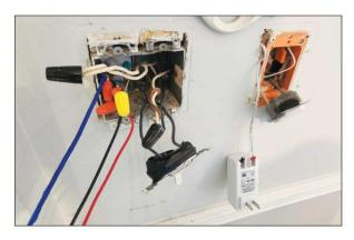
the receptacle. Instead, they twisted and capped the ground wire pigtail from the grounding screw in the metallic box to the neutral wire.
